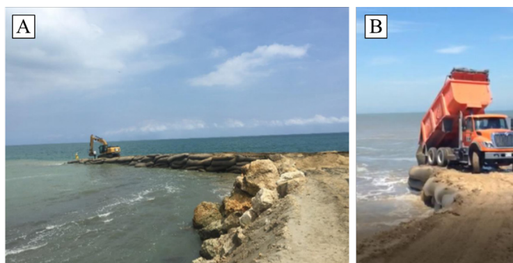
Figure 8. Submerged wall construction process (A and B)
