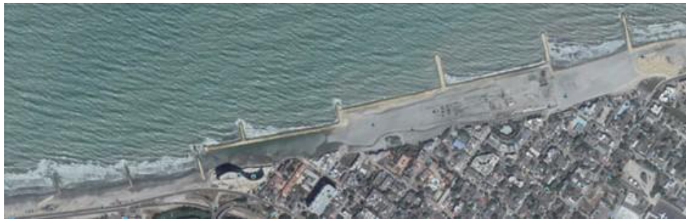
Figure 10. Satellite Images of construction. February 2012. Construction of seawalls (30)
