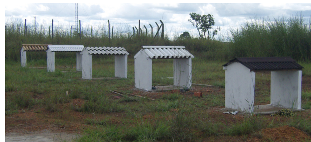
Figure 1 Reduced models with the respective roofing installed
